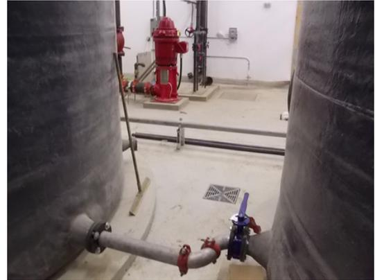
These tanks were lined with AOC's Vipel F010-H2O vinyl ester coating system, an NSF-certified resin that made this project possible for Structural Composites.
