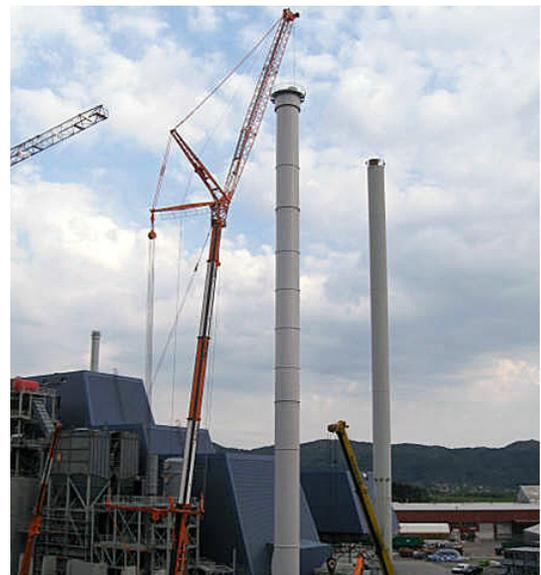
The composite liners were installed in a combined steel housing that was shipped to the plant site.
