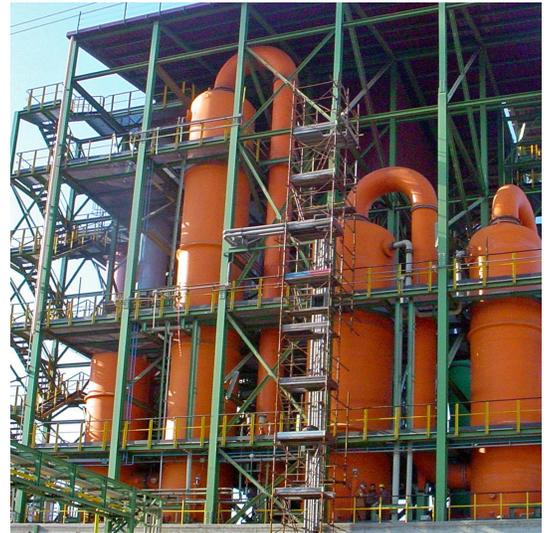
A large scrubber system at a major manufacturing site in Taranto, Italy, converts highly corrosive waste fumes into emissions that meet Europe's strict air quality standards. To ensure high performance and durability, scrubber components were made of fiber-reinforced polymer (FRP) composites based on Vipel resin technologies from AOC.
